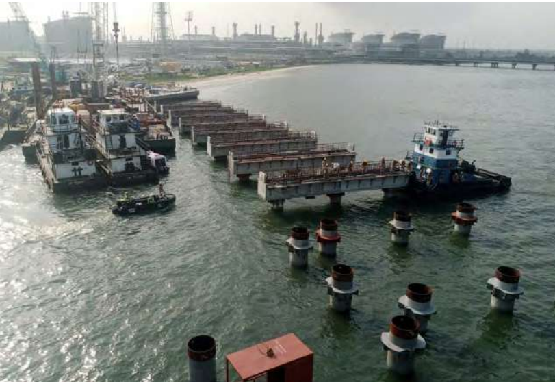
LNG project | Trevi Foundations Nigeria, Bonny Island, Nigeria
